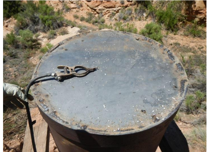
Sealed vent shaft
