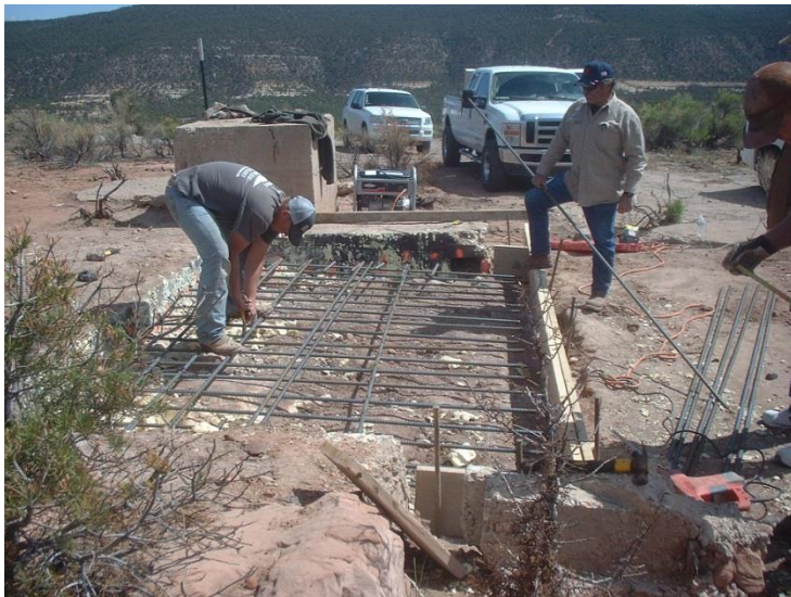
Rebar concrete reinforcement over PUF in access shaft
