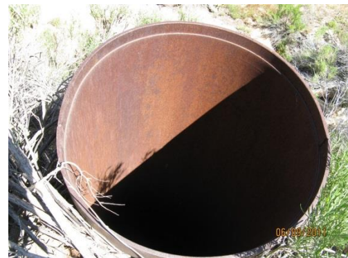
Uncovered ventilation shaft
