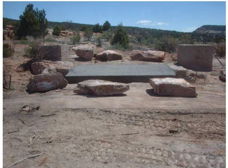
Completed construction with concrete cap and rock barrier
