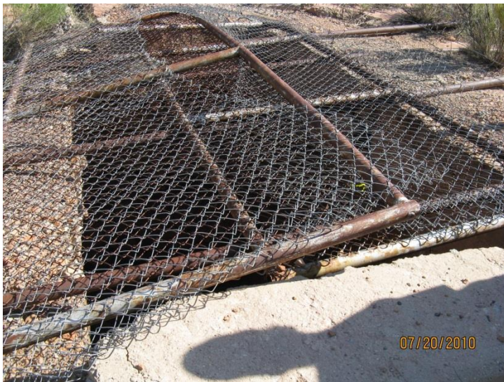
The shaft with temporary chain link barrier.
