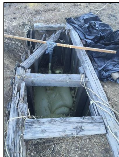
Below: Polyurethane "puf" is used to fill this hole.
