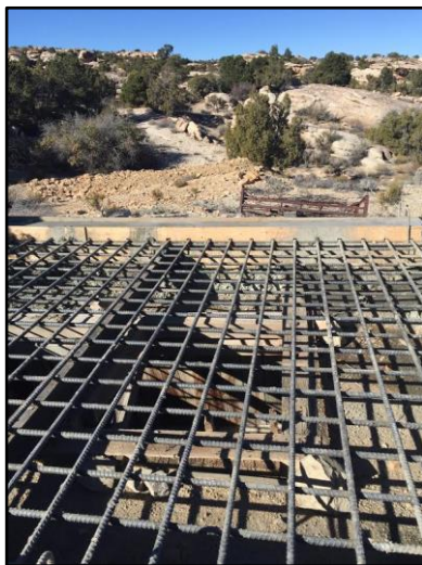
Left: Grates allow bat access while keeping people safe
