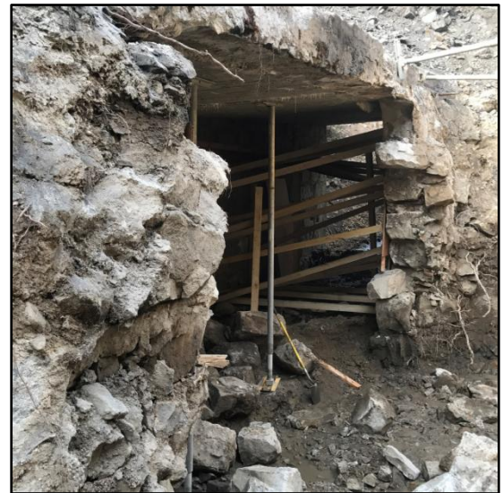
Above: (Pre-construction) Partially collapsed culvert wall Below: (Post-construction) Repaired culvert wall
