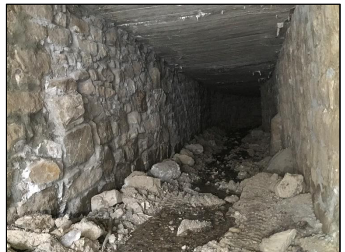
Above: (Pre-construction) Partially collapsed culvert wall Below: (Post-construction) Repaired culvert wall
