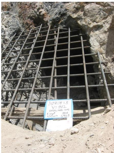
Site 3081813VO002 with rebar grate closure.
