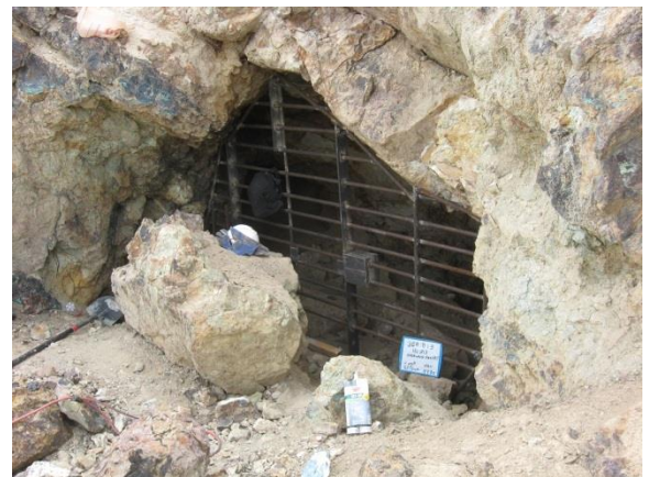
Site 3081813HO013 with bat gate closure.
