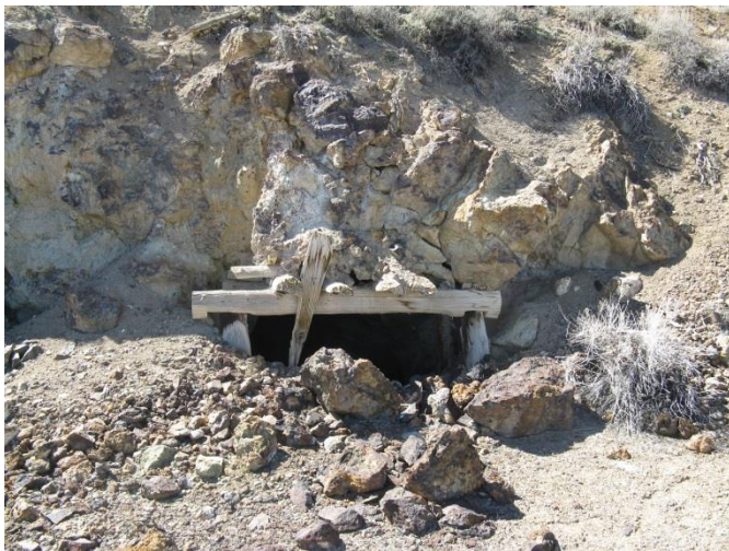
Site 308181310005 before closure with hazardous boulders perched on the old timbers and after closure with the boulders scaled down and a bat gate installed inside.
